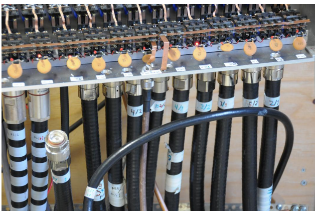
View in front of Veijo. Some of the antenna cables had loose connections, somewhere, and this caused obscurities at the station.
