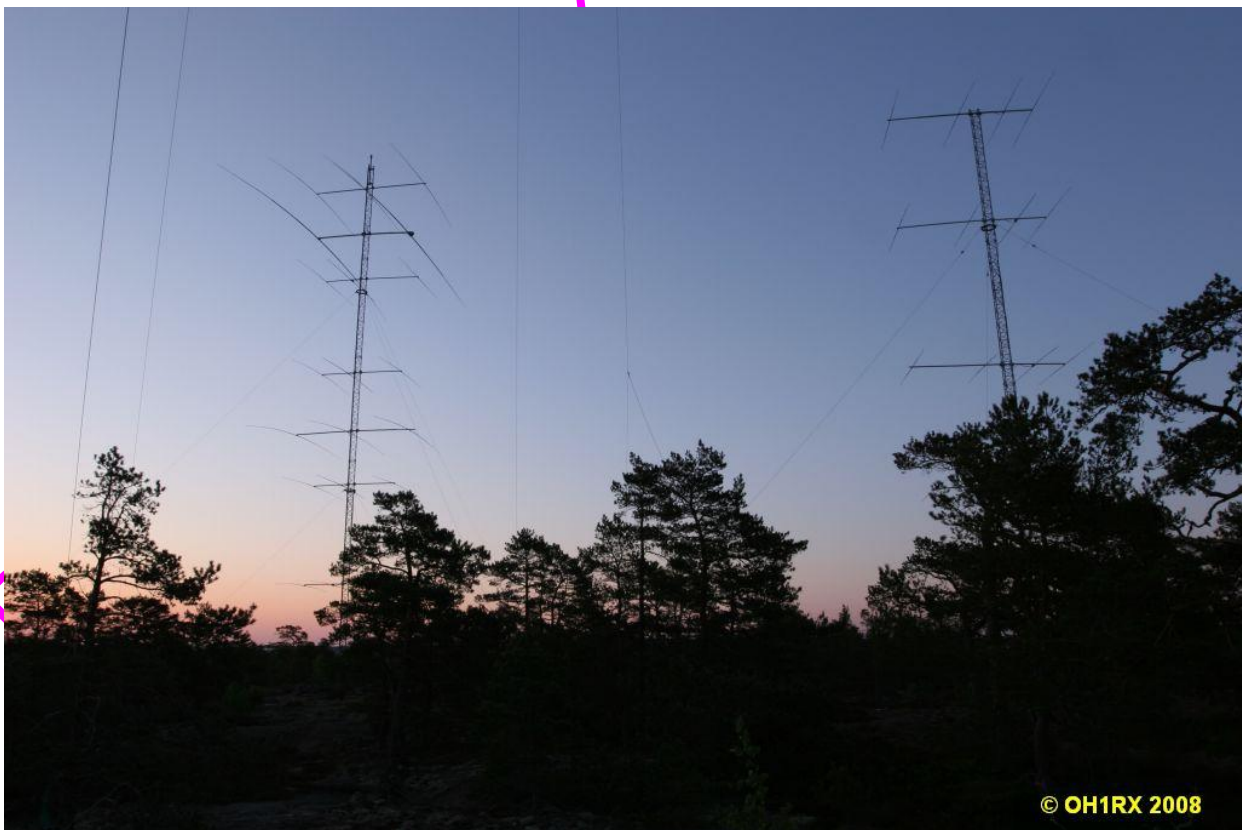
OHØZ at sunset, 23.5.2008, 10m tower on the right.
